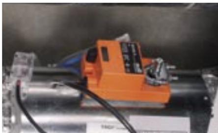
The VAV units from Trox are equipped with VAV-Compact controllers NMV-D2M from Belimo. They receive their setpoint values digitally, directly via the MP-Bus.
