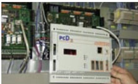
For each storey, one DDC controller of the PCD2-series with a MP interface from SAIA-Burgess operates 6 MP-Bus lines each, to which up to max. 8 VAV controllers NMV-D2M can be connected.
