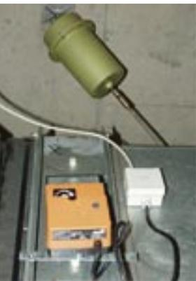
The existing ventilation plant room in the attic is still partially equipped with pneumatic actuators. These will now be gradually replaced by electrical direct coupled actuators from Belimo.
